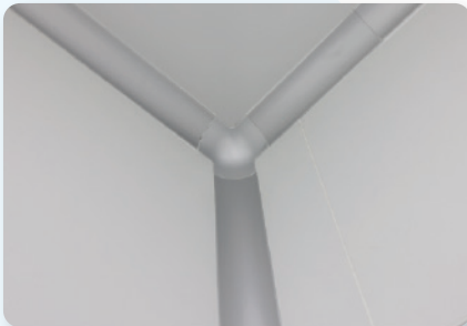
Wall to ceiling connections
