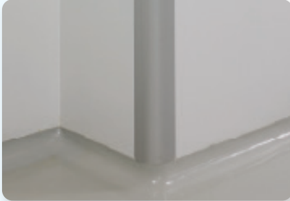
Floor to wall connections
