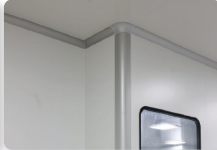
Wall to wall connections
