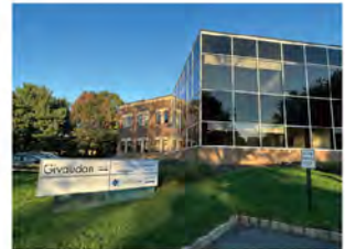
New Jersey Site
